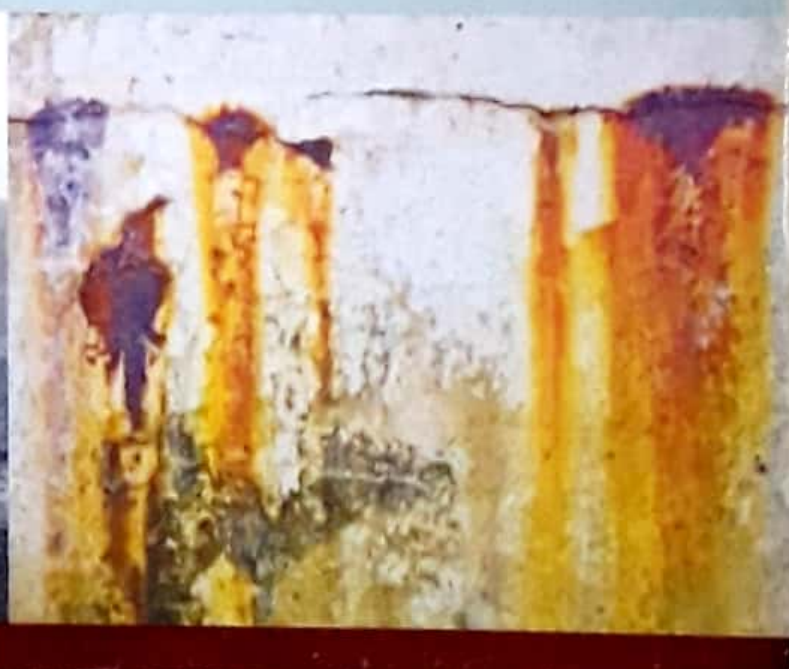
Single or Multiple Cracks
